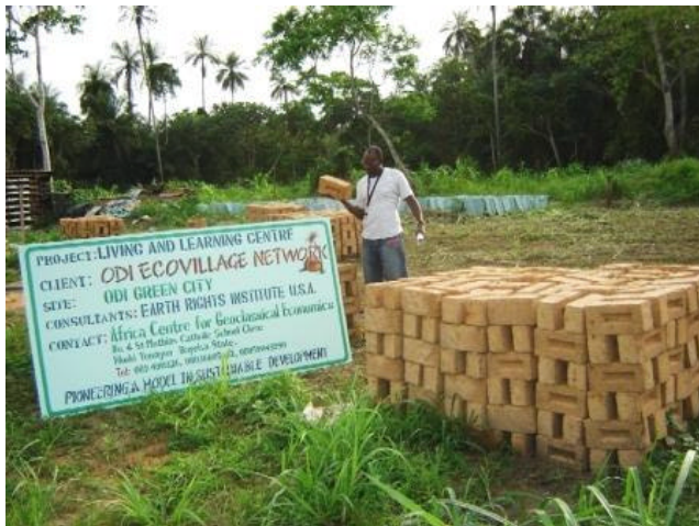
Gordon Abiama on site during construction (April 2006)
