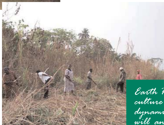
Site Clearing / Preparation
